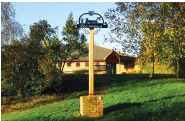
The Village Hall (built in 2000) with village sign in front
